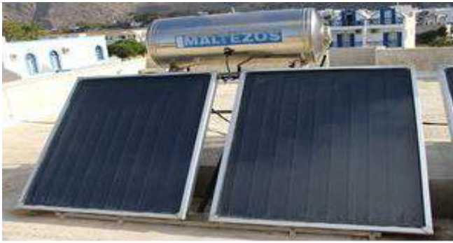
Fig.1 Simple heat absorber panel
