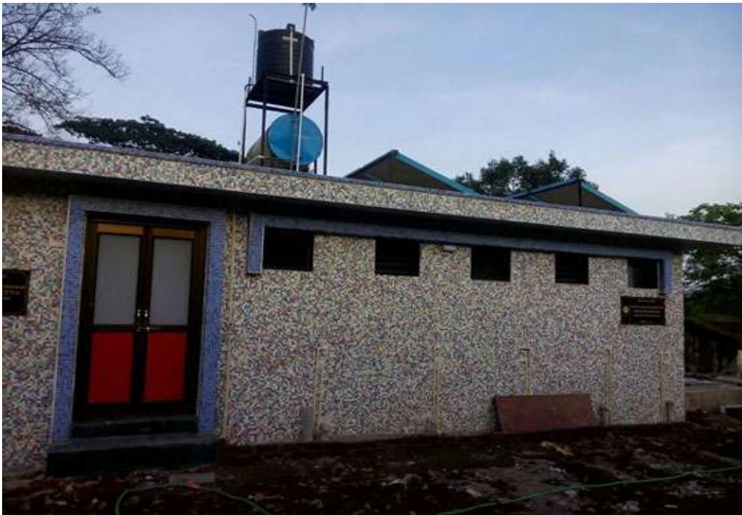
Toilets made for Villagers
